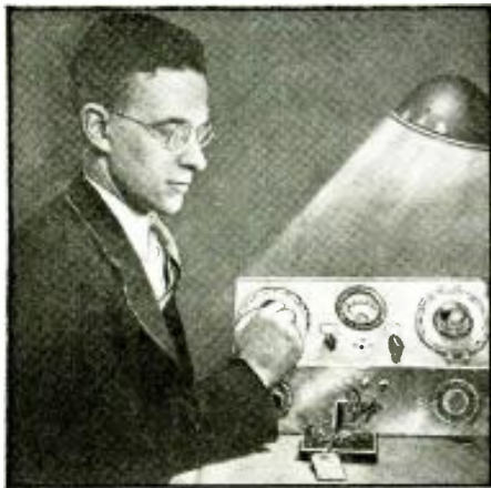
Fig. A. Mr. Lyons with his coil and condenser test unit, checking a sample coil. While "Q" and "absolute gain" are important items in coil design it is sufficient, in production coil testing, to have a device such as this Comparometer (as the author calls the unit) which is calibrated in "per cent gain" only.
